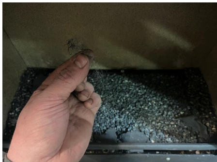
Fig.12 Add slate chips
